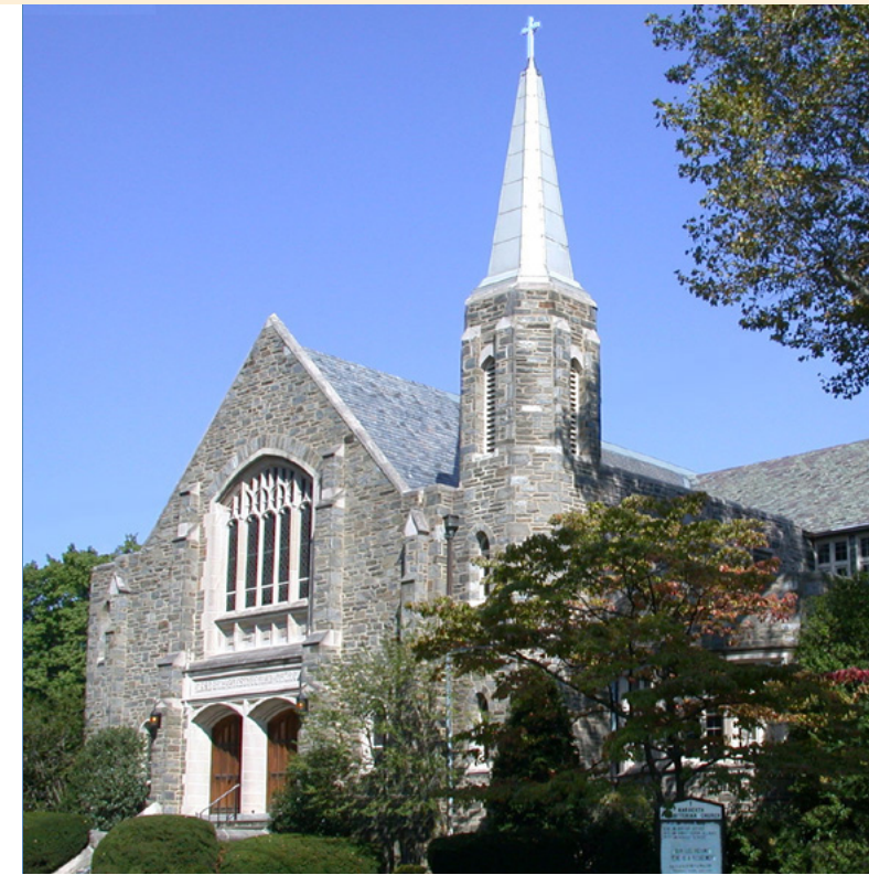
Exterior of Building
