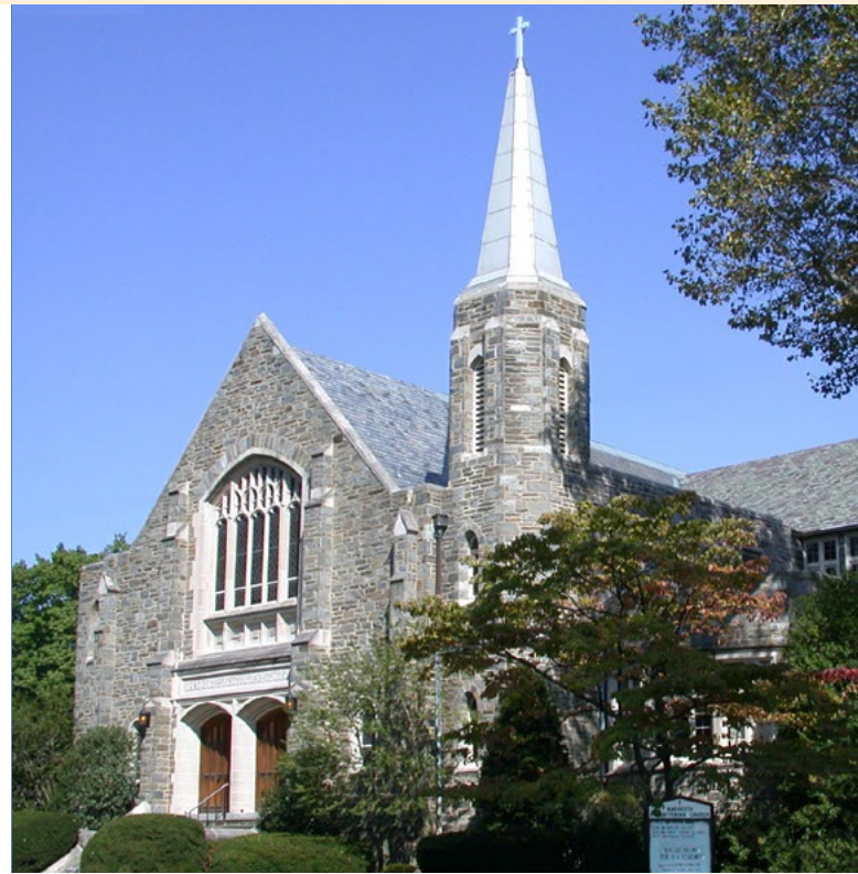
Exterior of Building
